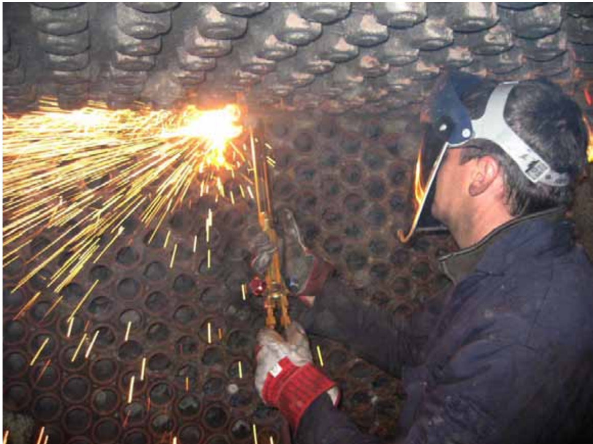
Philip Lewis cutting tubes in the J27 firebox on 22 nd September (Richard Pearson)
