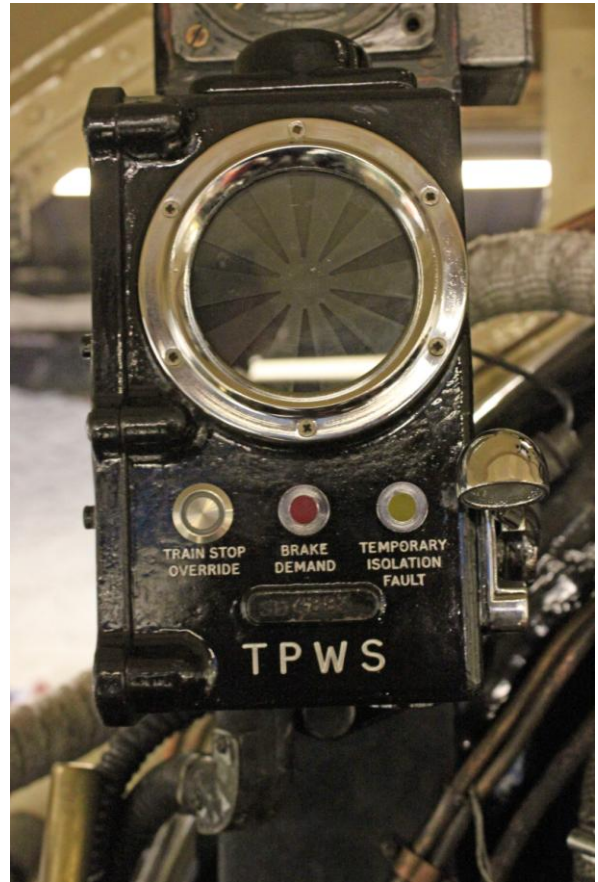
The 'new' AWS/TPWS indicator; acknowledgement is now via the silver handle to the right of the temporary isolation button
