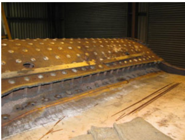
Welding in progress
