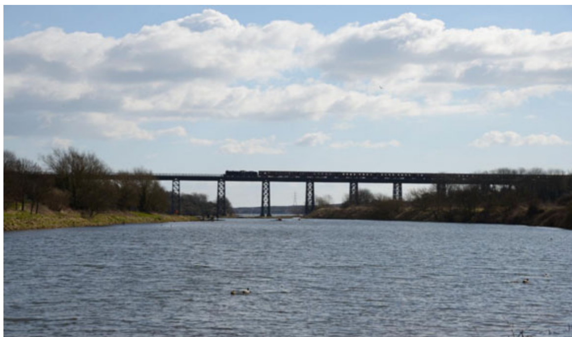
62005 stands on North Seaton viaduct on 30 th March (John Hunt)
