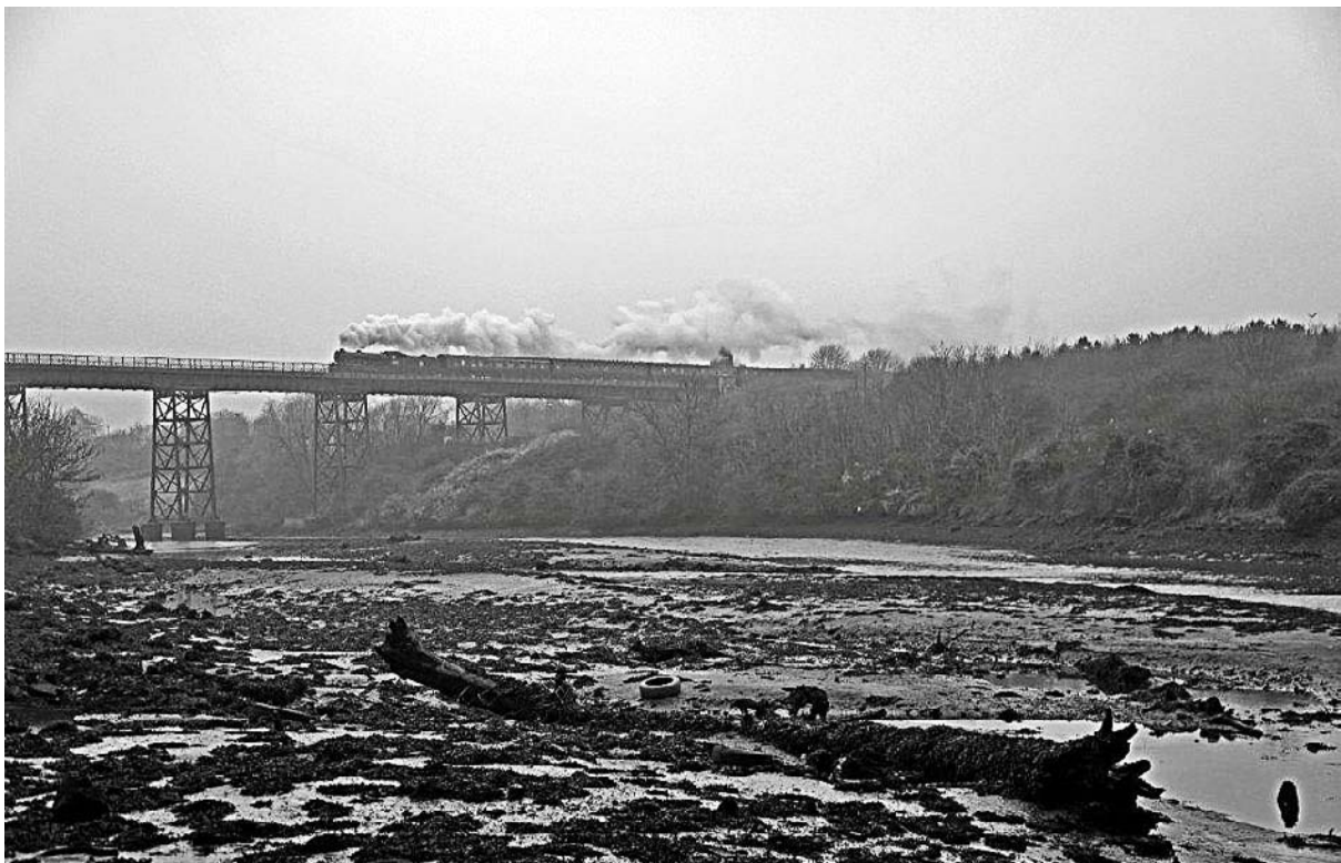
This fine monochrome image sums up the weather on the day, as 62005 heads south across Bedlington viaduct over the River Blyth (Ben Collier)
