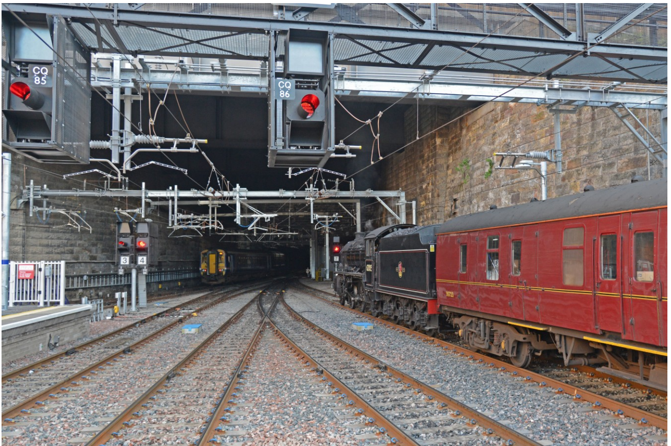
The K1 awaits departure from Glasgow Queen Street, a station much changed from steam and even diesel days, with the onset of electrification, track renewal and platform improvements. Only the 1½ miles of 1 in 41 to Cowlairs remains the same! (John Hunt)
