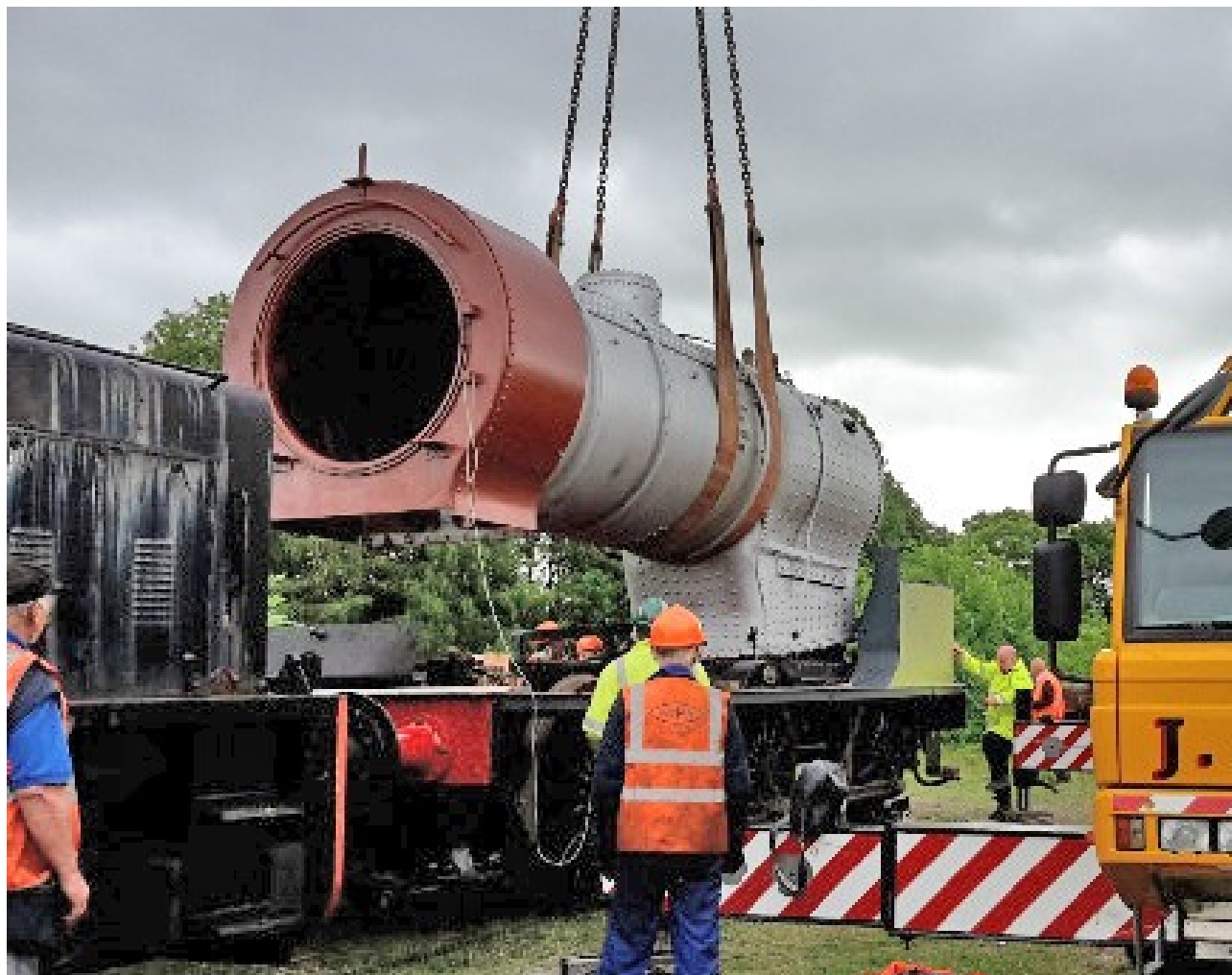
The J27 boiler is lowered into the frames at Hopetown on 23 rd June (Nigel Hall)
