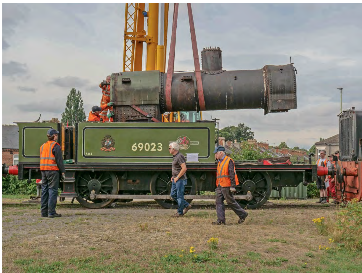
The J72 boiler lift on 6 th August: in the foreground are James Percy, Fred Ramshaw and Steve Hyman (Peter Giroux)
