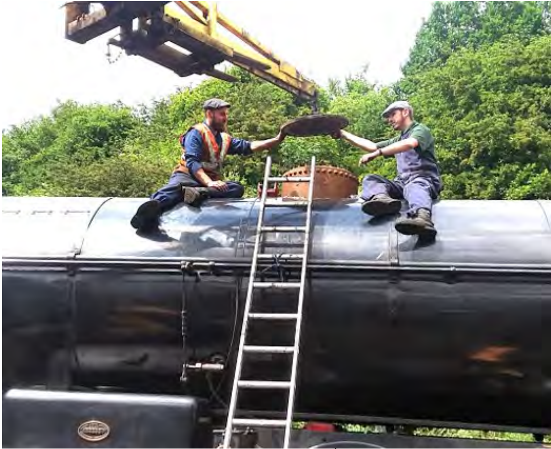
The Q6 dome cover being replaced on 6 th August (Bill Dobson)
