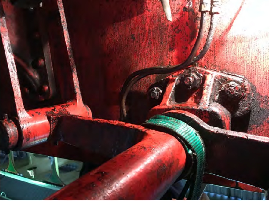
View of the engine way shaft bearing block. Note that the 3 fixing bolts are at the bottom of the picture (Ian Pearson)
