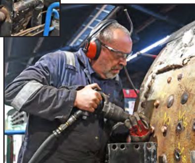
Andy Harper, ex NYMR boiler smith, but now working for NESL, beading over the two rows of new copper stays on the J27's backhead (top photo) and giving similar treatment to a fewer number of stays on the RHS, pictured on 15th July (John Hunt)
