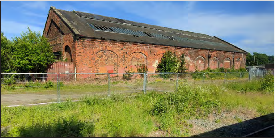
The 1861 building photographed from a passing train on 20th June (Maurice Burns)
