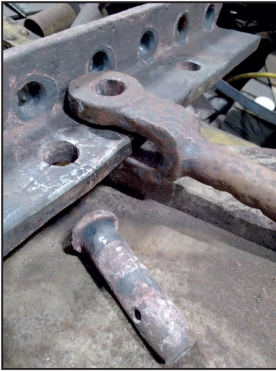
The fractured tube plate longitudinal stay strap with one of the short longitudinal stays and the securing pin. In addition to the fracturing in the strap, seen radiating from the hole to the left of the stay, corrosion fatigue can be seen in the stay (Paul Hutchinson)
