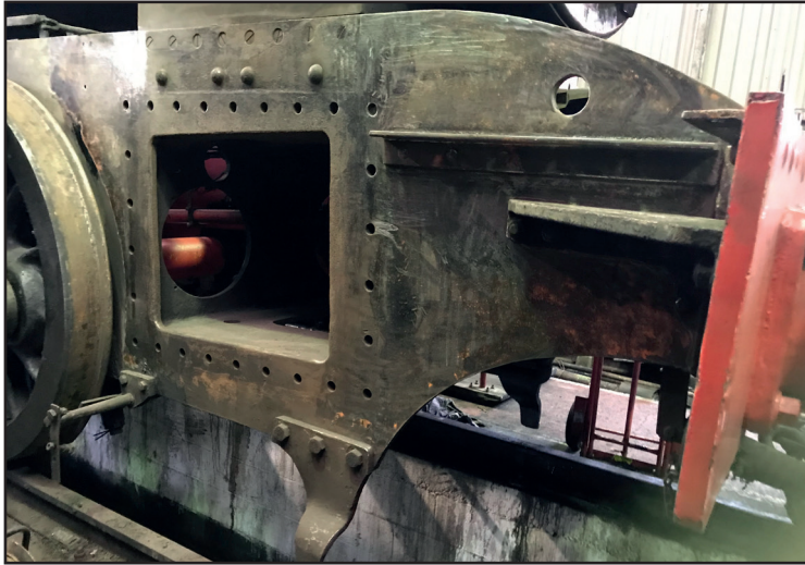
A view showing where the cylinder has been removed, and the frames cleaned ready for painting (Ian Pearson)
