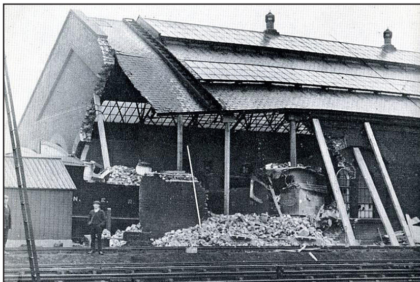
The 1861 locomotive shed at Darlington after the accident, with the pilot engine parked at 45 degrees across the line. The new brickwork is still visible today.
