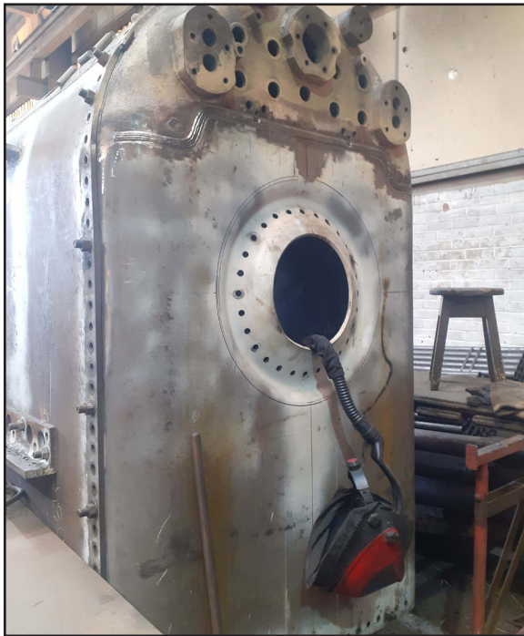
The new three-quarter steel outer backhead welded into place (Dave Pennock)
