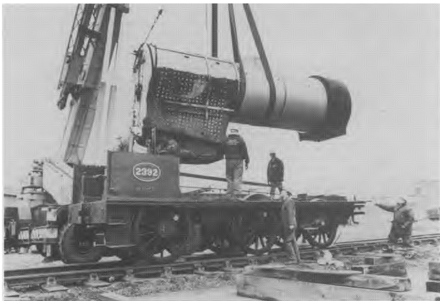
ICI riggers lift the P3's boiler at Wilton on 11th November 1993 (Maurice Burns)
