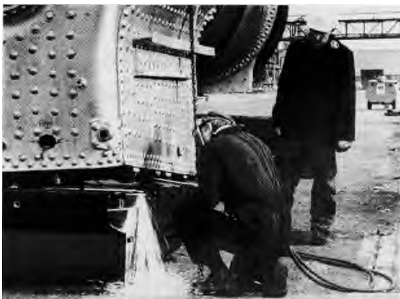
Minor adjustments being made to the new hopper ashpan by Maurice Burns at Wilton on 21st November prior to fitting to the firebox; Richard Pearson looks on.
