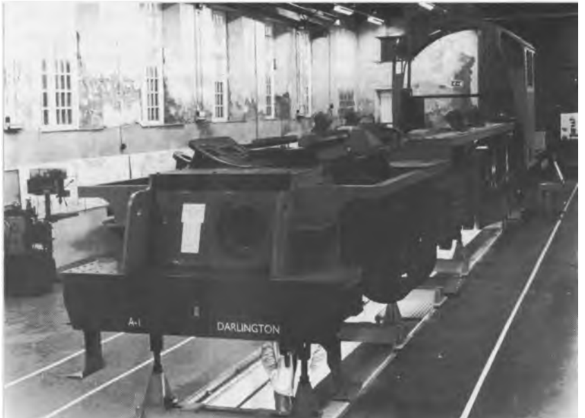
The new A1 60163 inside the works on 20th April (John Hunt)
