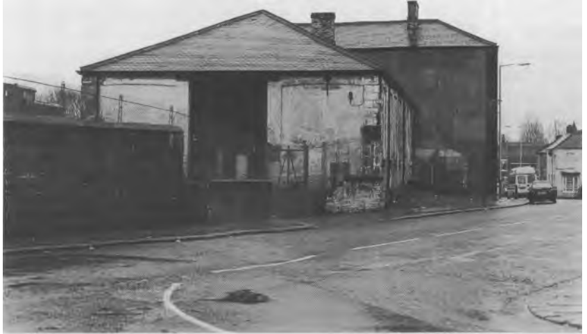
The west end of the S&D Hopetown Carriage Works at Darlington. After demolition of the wall in the foreground, locomotives would enter the building through the double doors (John Hunt)
