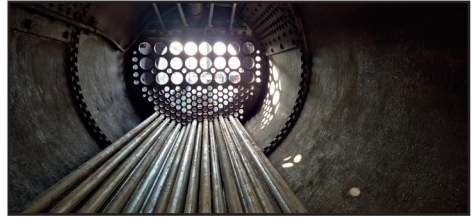
The view from the firebox and looking towards the front tubeplate with the first of the small tubes in place on 25th November. All the small tubes were in place by the 27th and a start made on expanding them (Rowland Bingham)
