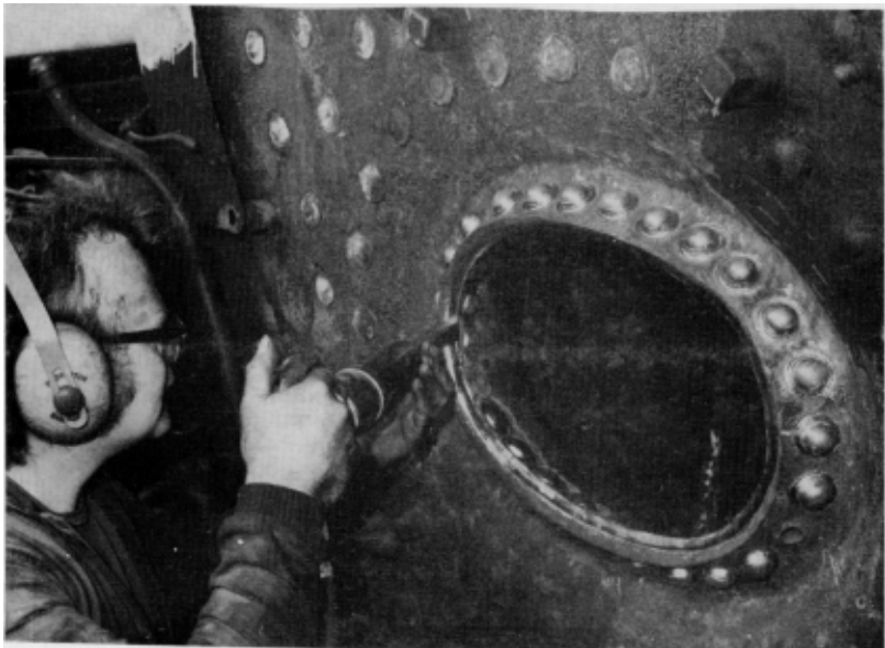
S.V.R. boiler smith Graham Beddoes tooling the firebox mouthpiece on the Q7 0-8-0 No.63460 following the fitting of new rivets on 21st June. (John Hunt)
