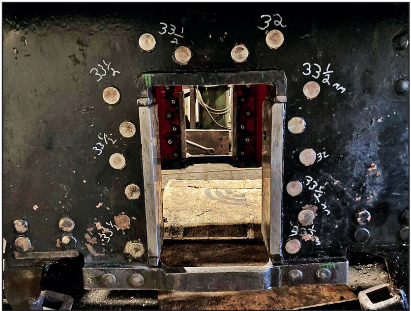
New fitted bolts fitted later the same day (Ian Pearson)
