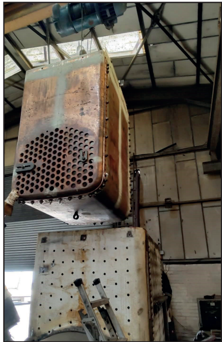
Pre stay hole drilling from Barney Casey during a previous offer of the new copper box to the outer firebox.
